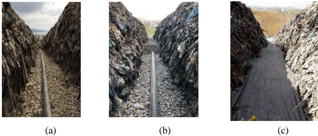
Figure 2. a, b, c) Installation of Rigol Lines in Harmandali RWSF
