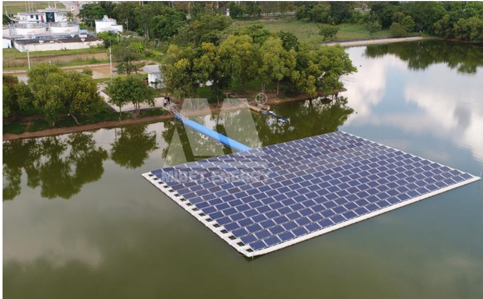
Figure 1. The floating solar system installed in Thailand [20]
